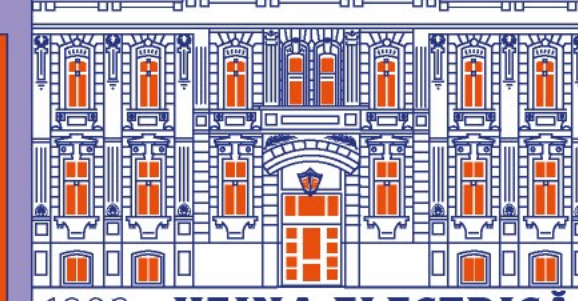
1892 - UZINA ELECTRICA ELECTRICAL PLANT
